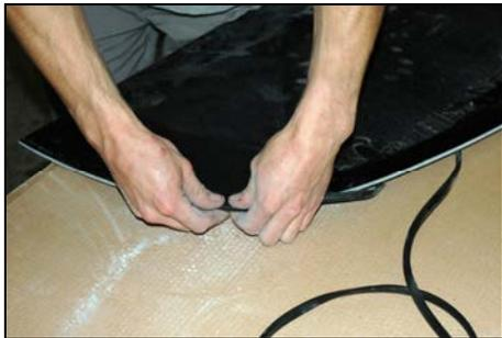
You should now apply the supplied edging strip to the edge of the panel. This makes the panel look neater and prevents water and dirt from becoming ingrained into the edge of the panel.
